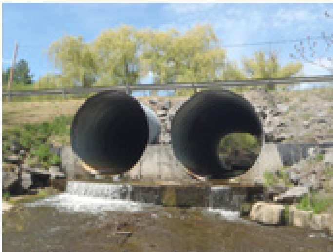
Fig 2: Removing barrier impacts on fish migration - replace culverts (Reproduced by permission of Engineering Ventures PC)
