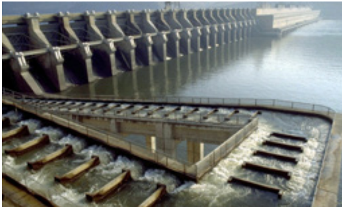
Fig 1: Removing barrier impacts on fish migration - install a Fish Pass (A Fish Ladder) at the John Day Dam on the Colombia River – source US Army Corps of Engineers)
